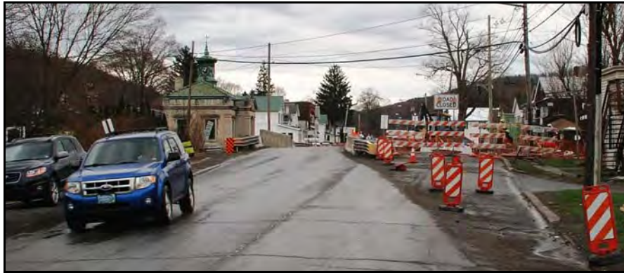
Route 11 Bridge Replacement
