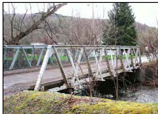
Johnson Street Bridge across Salt Lick Creek
