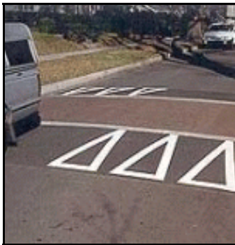
Speed table with stamped, colored concrete
