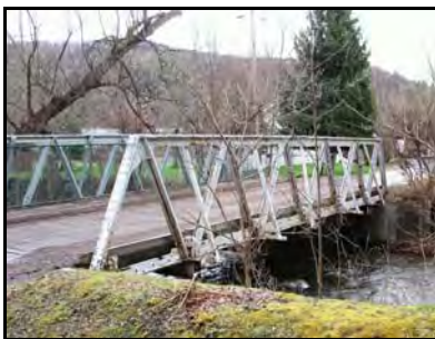
Johnston Street Bridge
